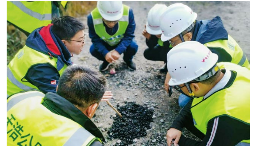
Workers of Suiyuan Expressway under Yuexiu Transport Hubei apply the hot-mixed recycling technology to the road surface
