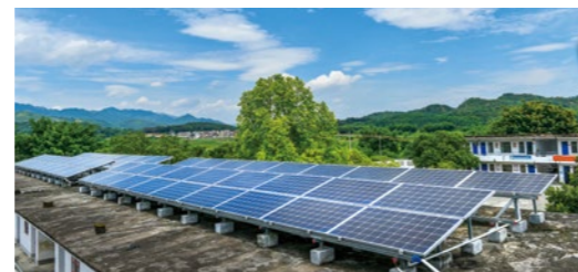
Rooftop solar PV panels in Chimi village
